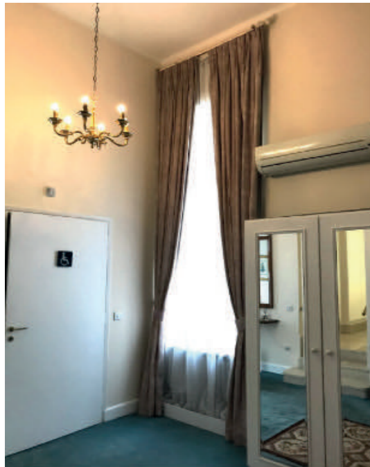
Existing womens bathroom room 51
