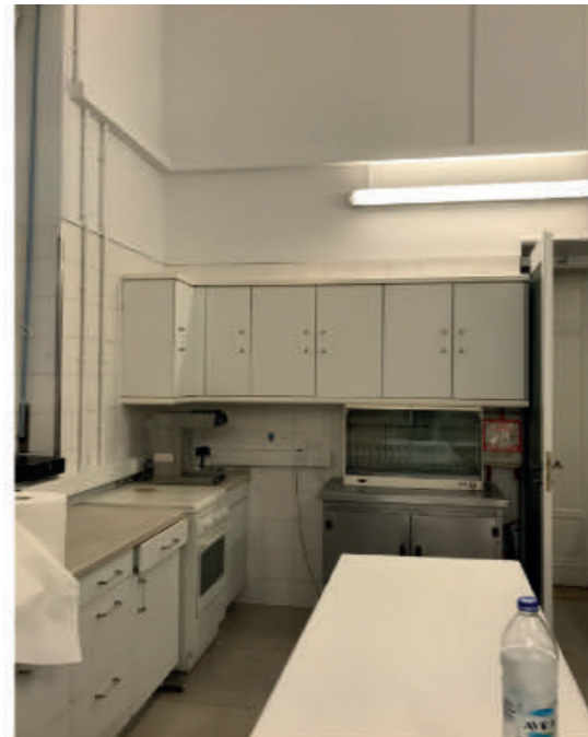
Existing servery room 41
