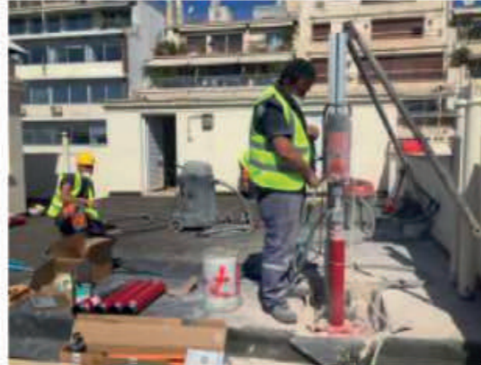
Hilti Drill in operation for vertical drilling in masonry wall
