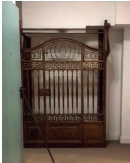
Existing lift frame in room 23
