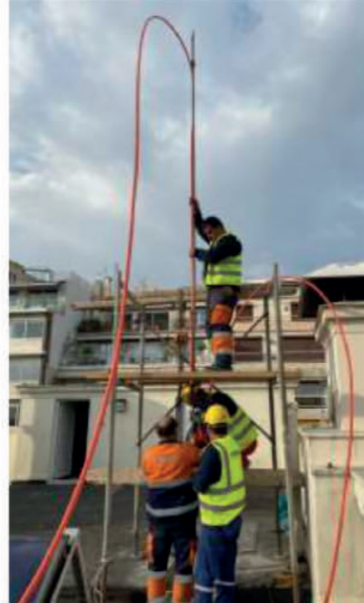
Installation of vertical rod
