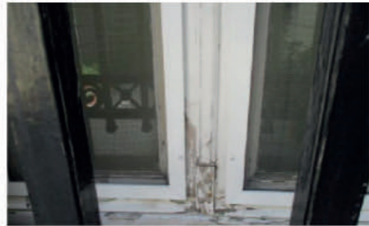
Spliced in timber repairs
