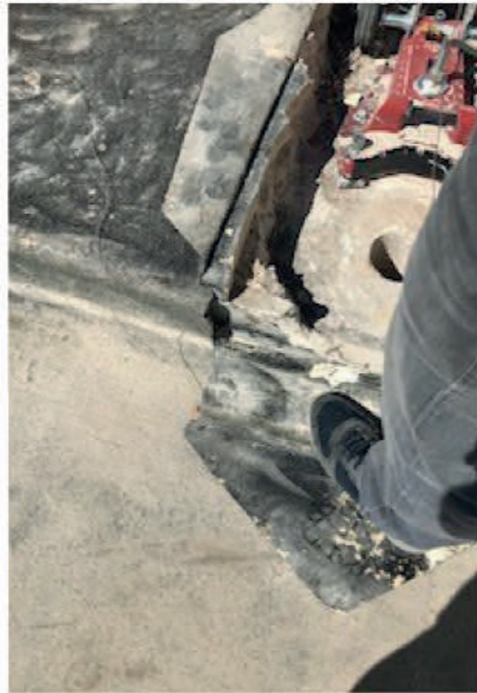
Roof showing core hole down into structure
