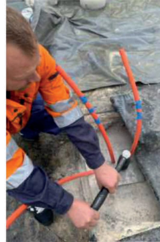
Post Tensioning of vertical rod
