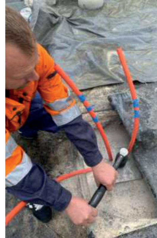
Post Tensioning of vertical rod
