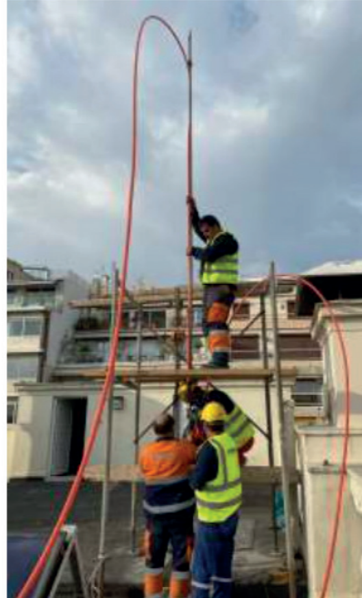
Installation of vertical rod
