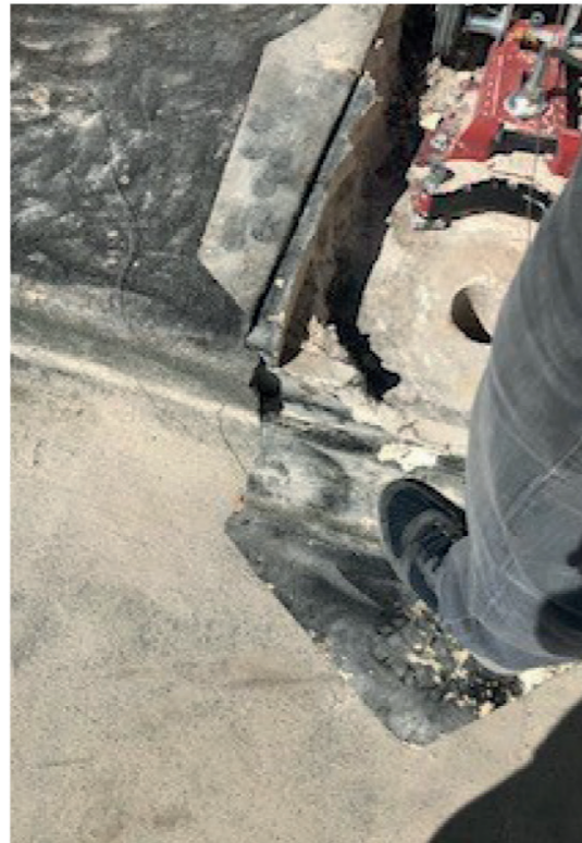
Roof showing core hole down into structure
