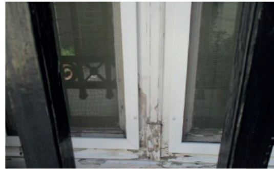
Spliced in timber repairs
