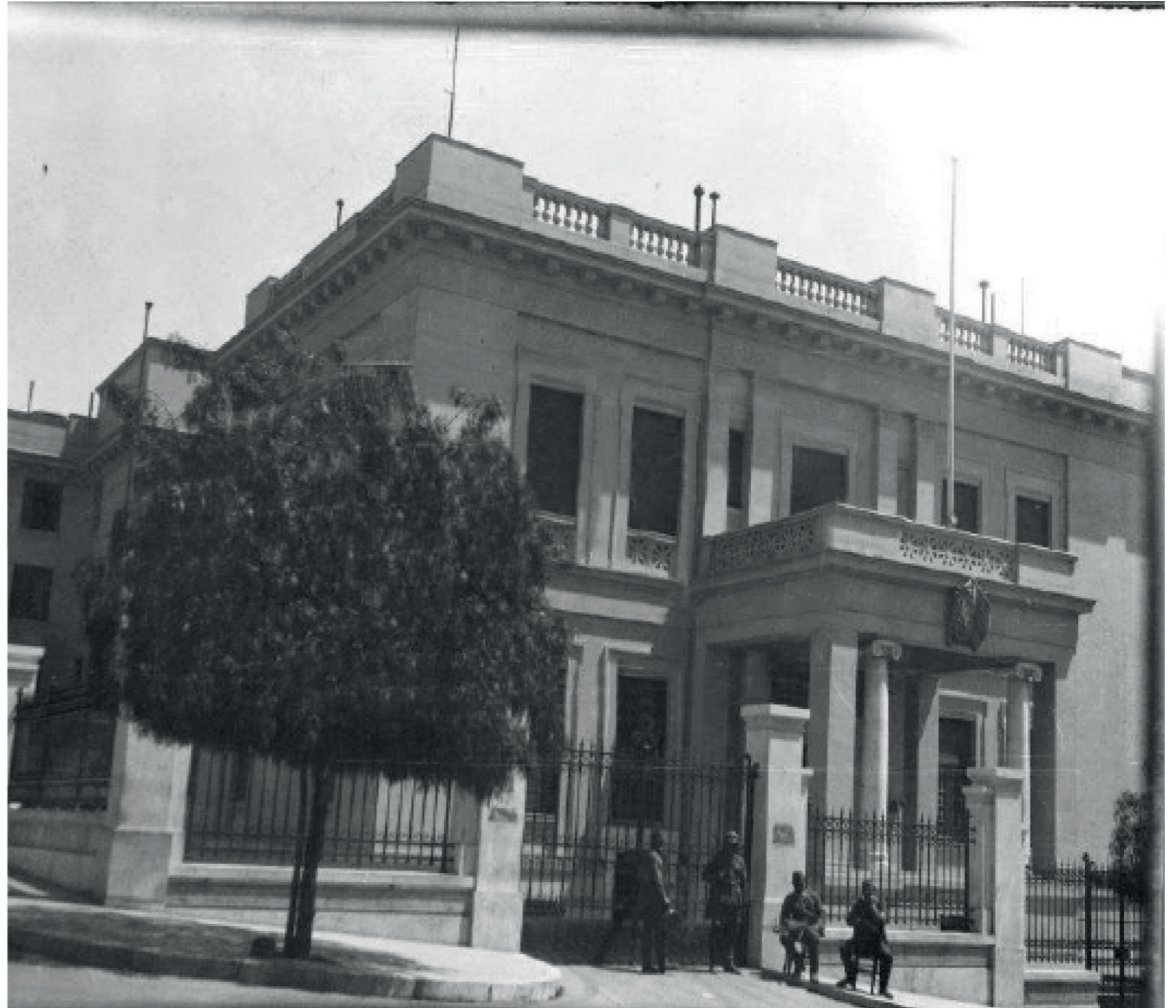
West view of the Residence from historical archives
