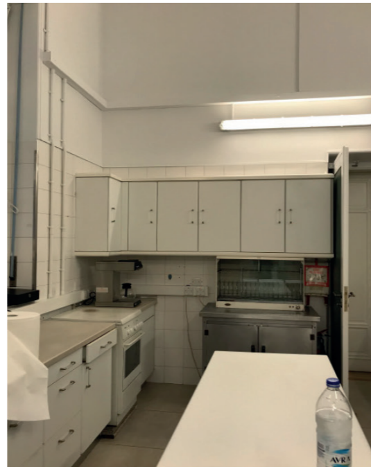
Existing servery room 41
