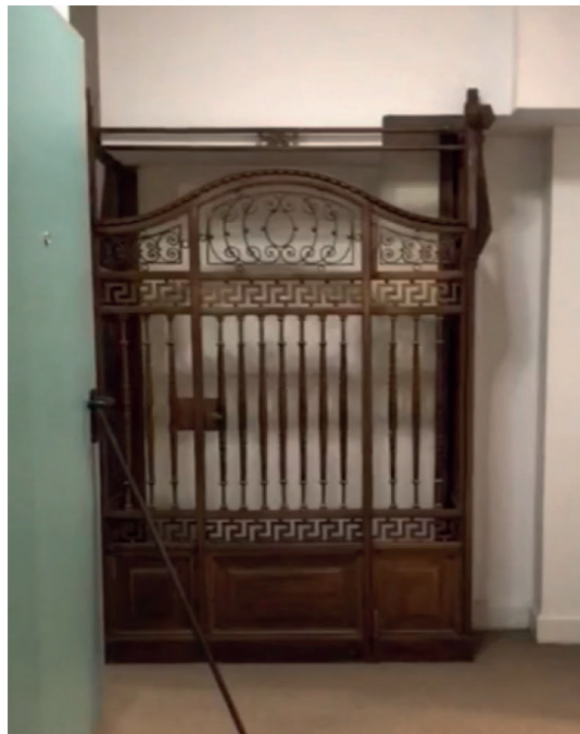
Existing lift frame in room 23
